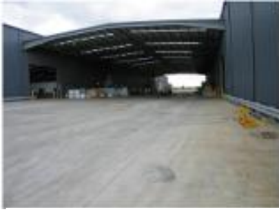
Awning area – No controls.
