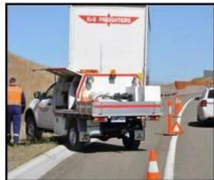
Using traffic bollards with triangles can create a visible barrier between workers and passing traffic.
